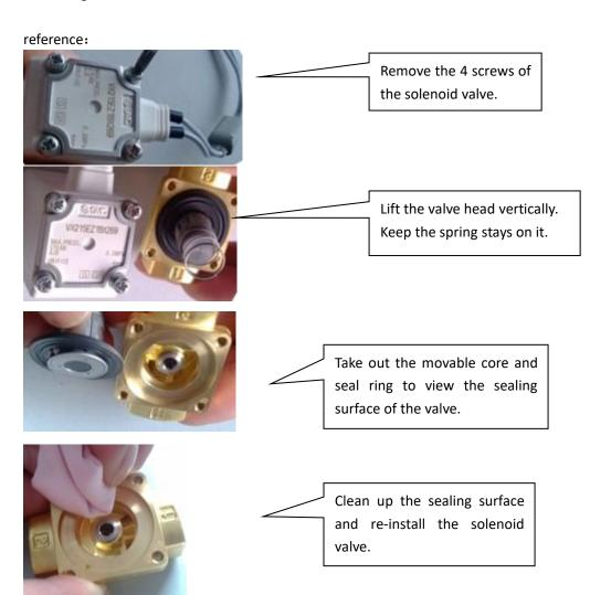
Thoroughly clean the parts after removing them. And then have a re-installation.
